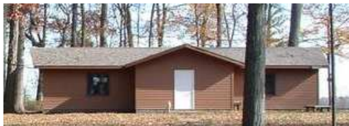
Cabin # 2 Nearing Completion
